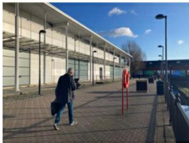
EXISTING BUILDING FROM DOCK EDGE
