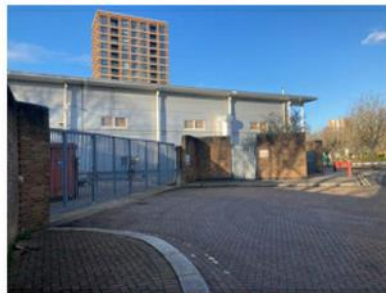
EXISTING SERVICING ACCESS
